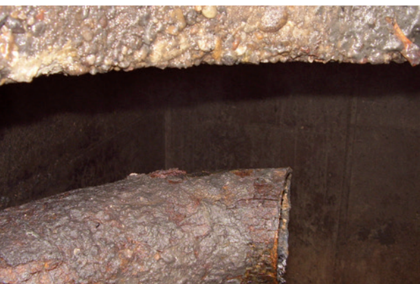
biogene Korrosion
