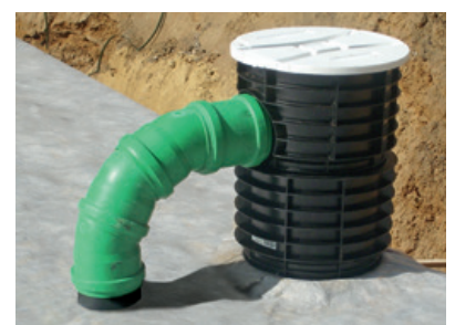
Creating a ventilation: A pipe elbow connects the upper part with the nozzle and the pipe connection adapter
