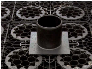
The pipe adapter is mounted in the previously cut out opening at the top
